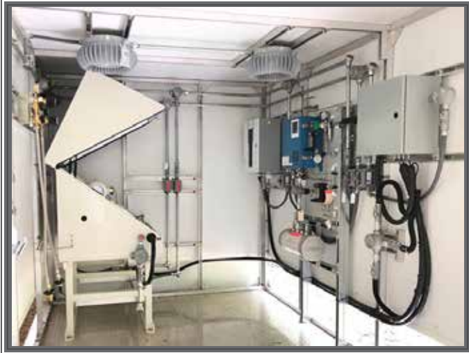
GC, Moisture Analyzer, Total Sulfur Analyzer, and Marshalling Panel.
