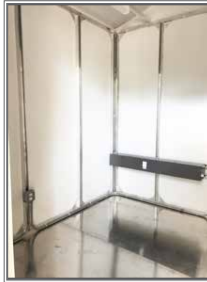
Skid Structure AL Floor with AL Unistrut Mounts
